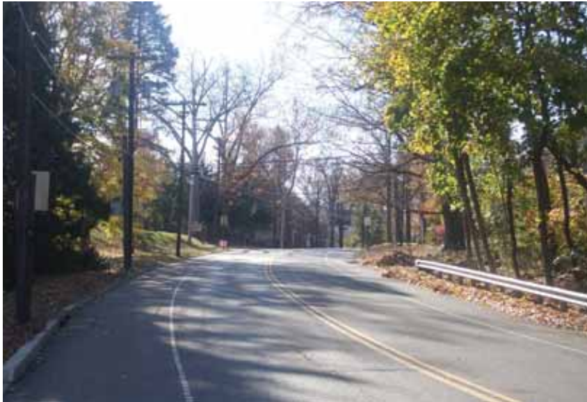
Existing conditions of Park Street Gateway
