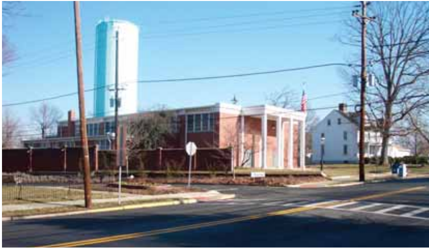
Existing Intersection at Union Street and Crosswicks Street
