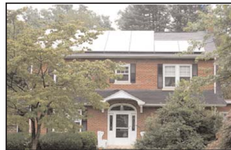
Solar panels at the Rossos' office/home
